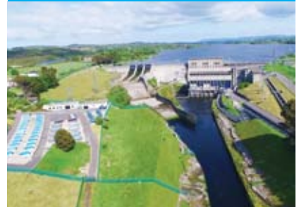
Hydro-Electric Station, Ballyshannon
